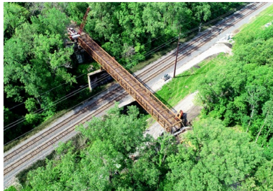
MCT Goshen Trail Bridge over active railroad tracks
